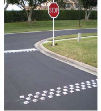
Botts Dotts and Raised Reflectors
